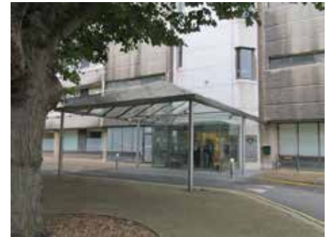
council office entrance.jpg
