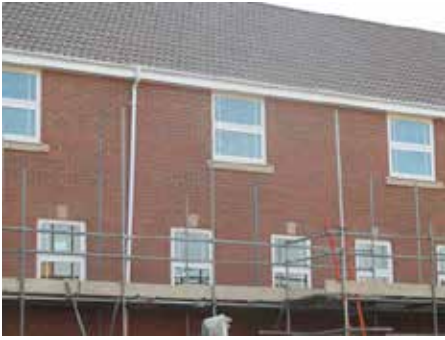
building construction site.jpg
