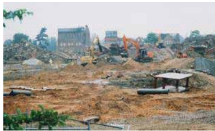
building site demolition.jpg
