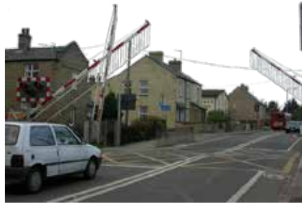
train level crossing barriers closing opening.png
