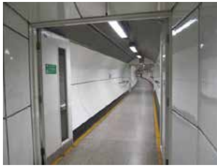
underground tube station platform corridor.jpg
