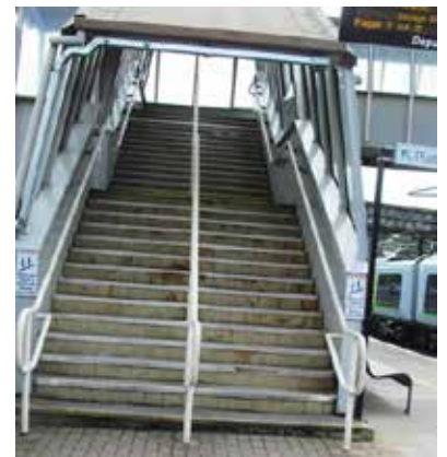
train station bridge steps.jpg
